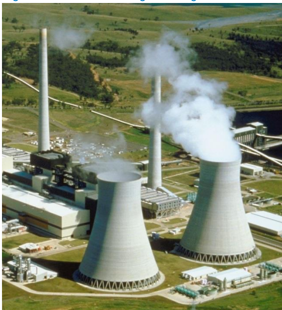
Figure 5.1: Natural draught cooling tower
