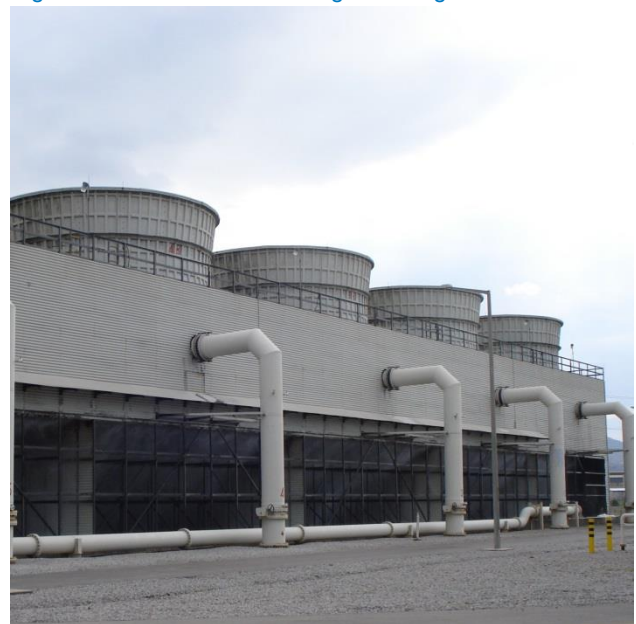
Figure 5.2: Mechanical draught cooling tower
