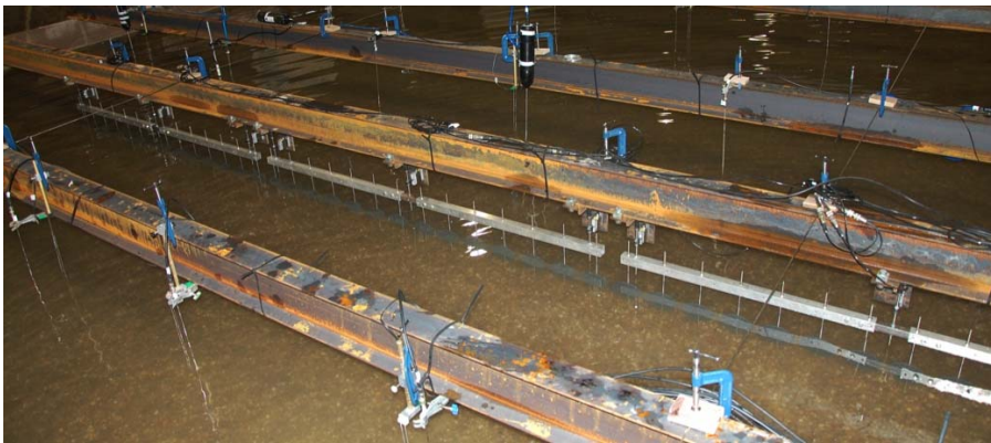
(b) 3 No. sections of 1.8 m long strip of discs, total 42 discs, installed at HRW CRF. 3 rd strip only part shown right hand side of image.
