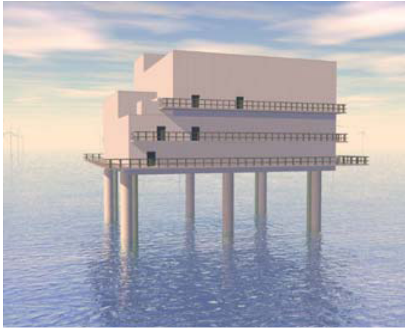
Fig. A13: Converter station at offshore wind farm, NordE.ON 2 Project where 400MW of wind power will be transmitted to Northern Germany, over 200km (Source: ABB website www.abb.com )
