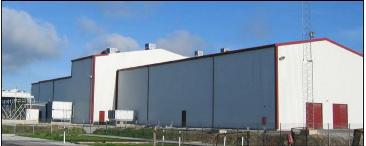
Fig. A11: Converter station of 350MW, \pm 150 kV Estlink VSC-HVDC transmission system based on two-level converter approach (Source: ABB website www.abb.com )
