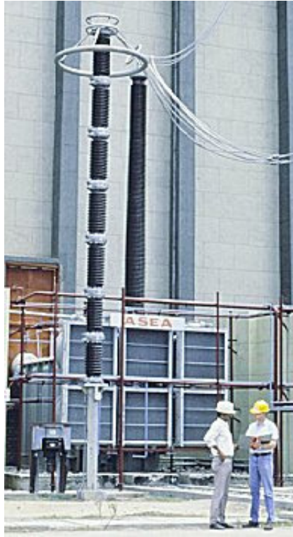
Fig. A7: Smoothing reactor (source: ABB website www.abb.com )
