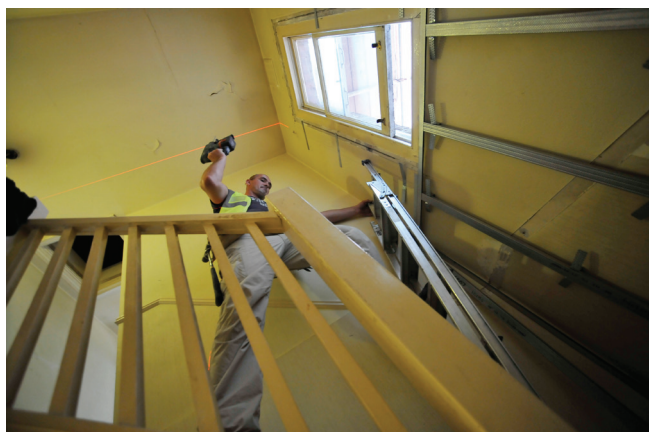
Figure 2. Retrofit work on site.
