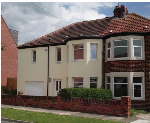
Figure 17. EWI installed on one side of semi-detached property. Source: www.building.co.uk
