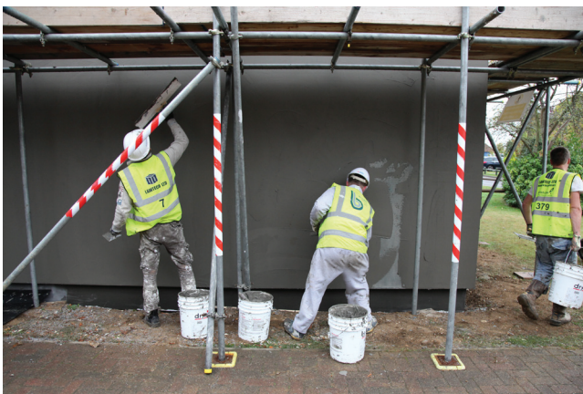
Figures 20 and 21. Resident engagement and retrofit work.
