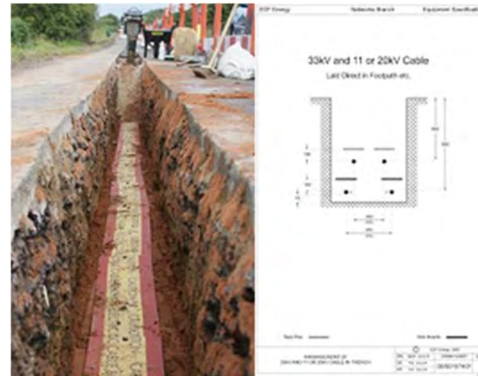
Figure 11-67 Example of a construction swathe for a land cable
