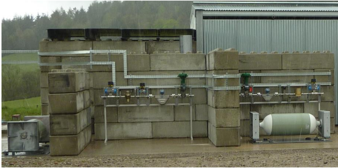
Figure 13: Gas delivery system
