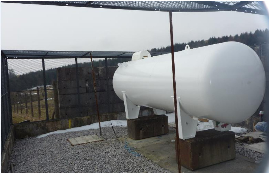
Figure 6: Butane supply tank
