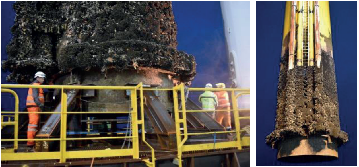
Figure 11. Decommissioned wind turbine showing hard fouling of the upper 2 to 3 m of the submerged structure.
