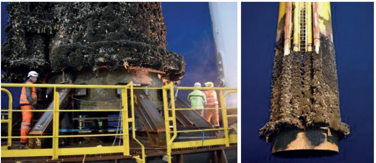
Figure 4. Decommissioned wind turbine showing hard fouling of the upper 2 to 3 m of the submerged structure.
