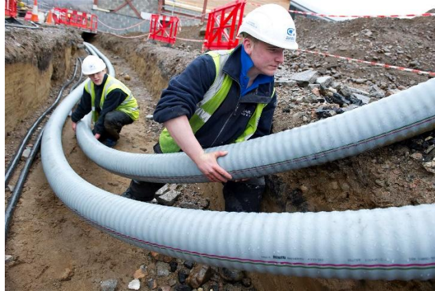
Figure 16: Trench-installed DH pipe (Source: Rehau UK)
