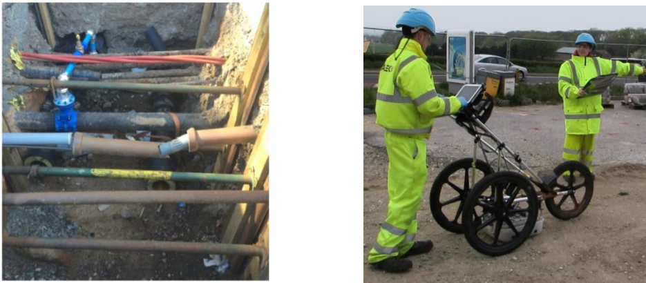
Figure 5: (a) congested DH route, (b) undertaking Ground Penetrating Radar survey 3
