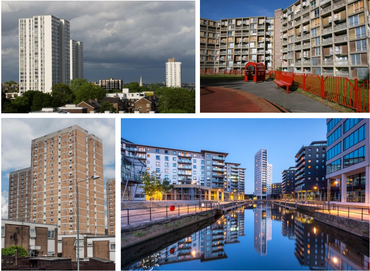
Figure 12: Examples of high rise flats.
