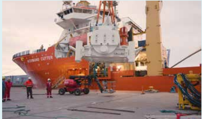
MeyGen Subsea Hub being lifted (Source: SIMEC Atlantis Energy)
