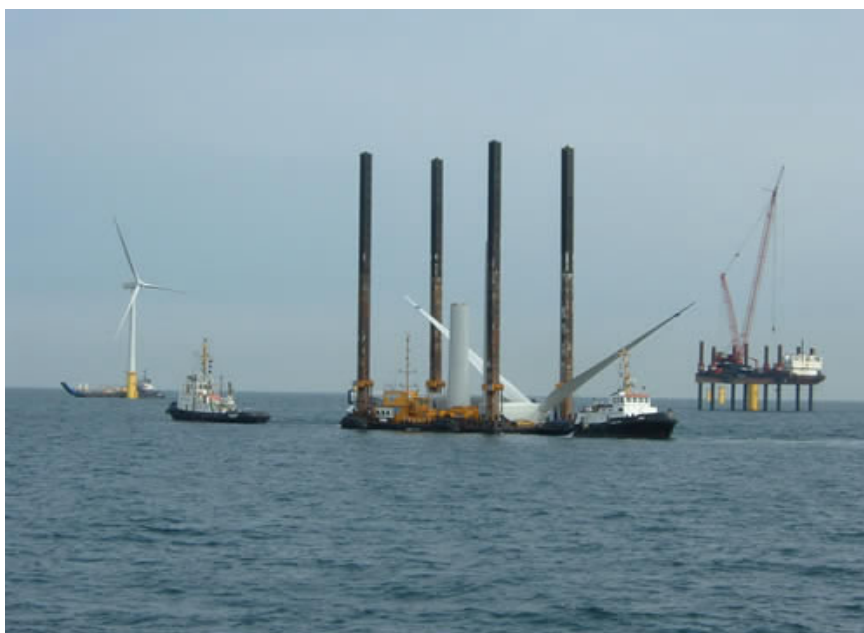
Figure 1 - Jack Up Installation Barge and Feeder Barge Constructing North Hoyle Windfarm
