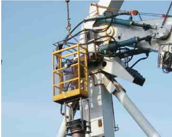
Figure 16: Bolting of arm to column
