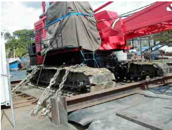
Figure 10: Crane seafastened for journey
