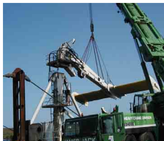
Figure 15: Arm/hydroplane section lift
