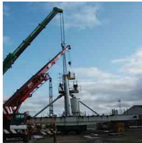
Figure 13: Preparing base section for lift
