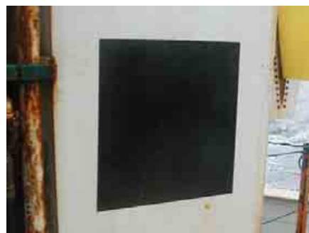
Figure 28: Image of main post taken to determine levels of marine growth during September 2003
