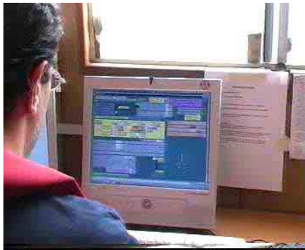
Figure 24: Main SCADA screen for PLC control (automatic mode)
