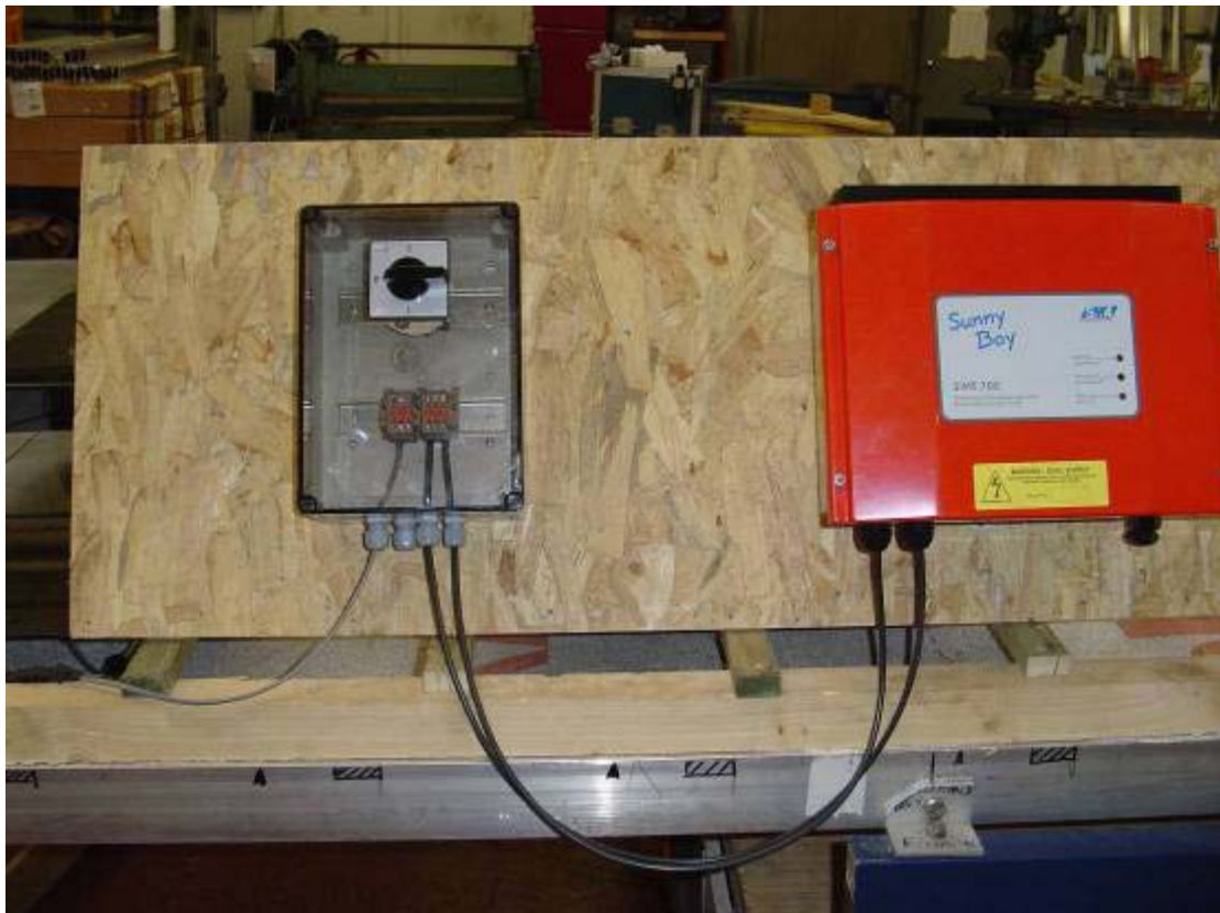
Fig AD. Connection to Marshalling Equipment.
