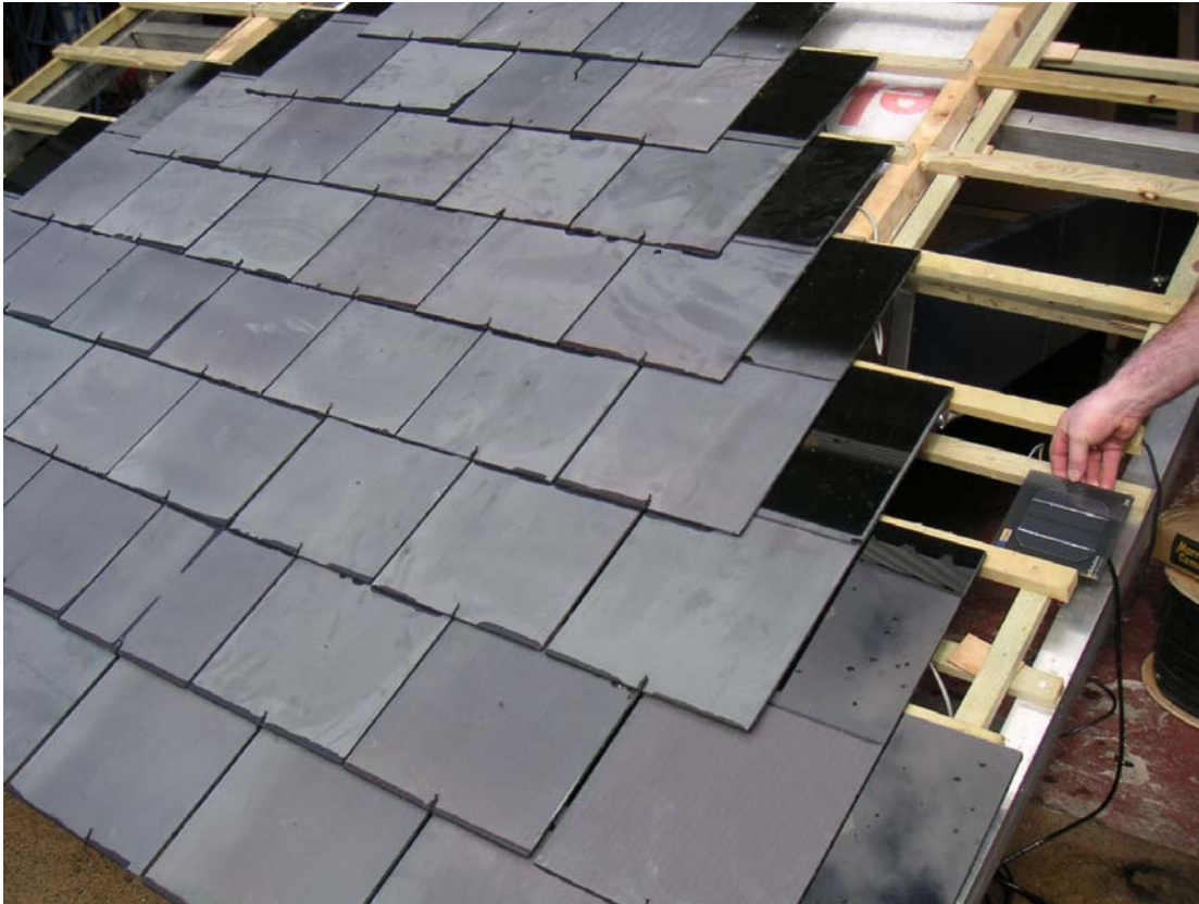
Fig B1. Roof Section under Test
