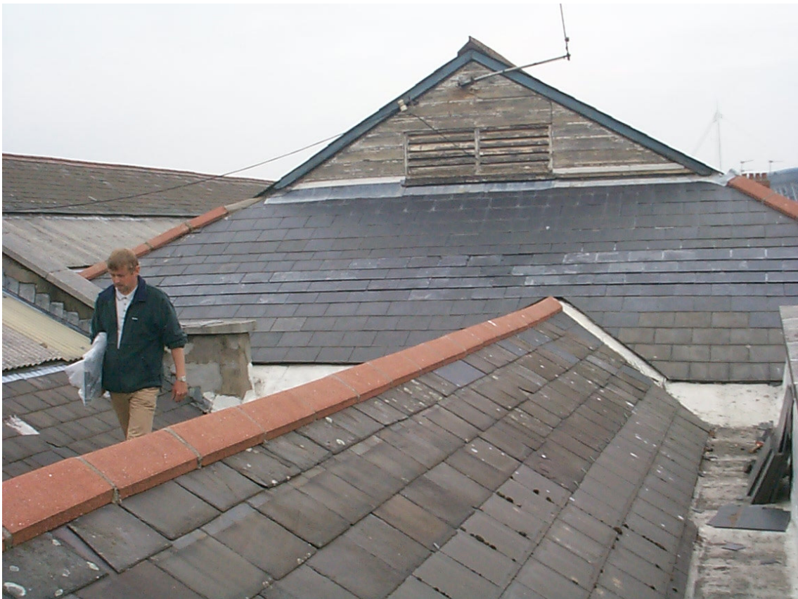
Fig C. Track 2000 Installation completed.
