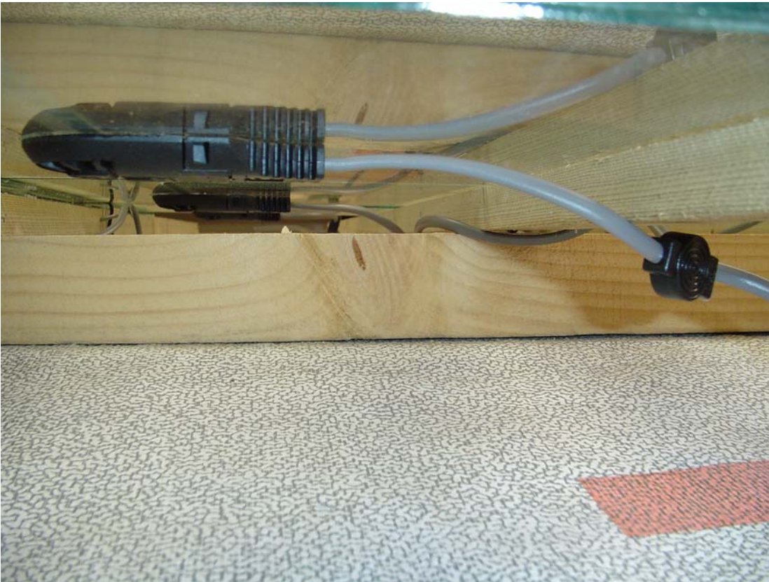
Fig BD. Under Slate Connection.
