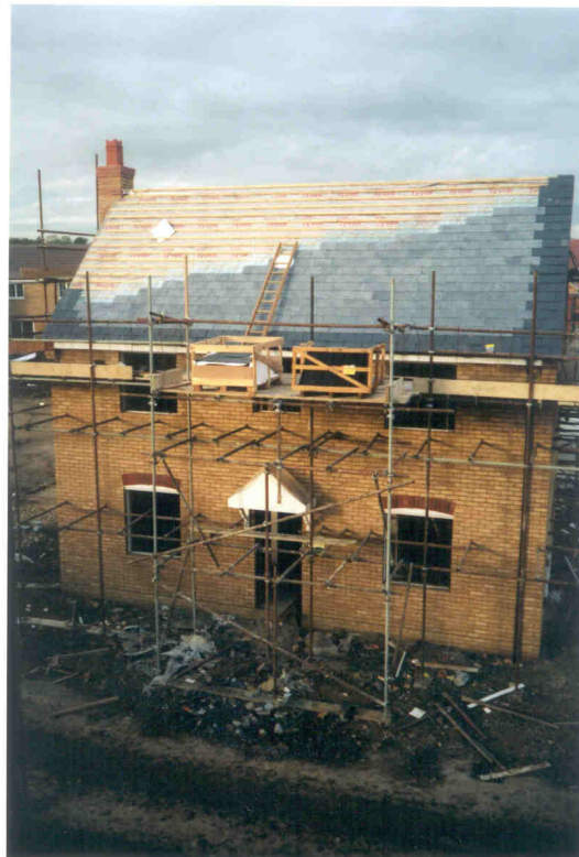
Fig E. Clapham Folly Work in Progress.
