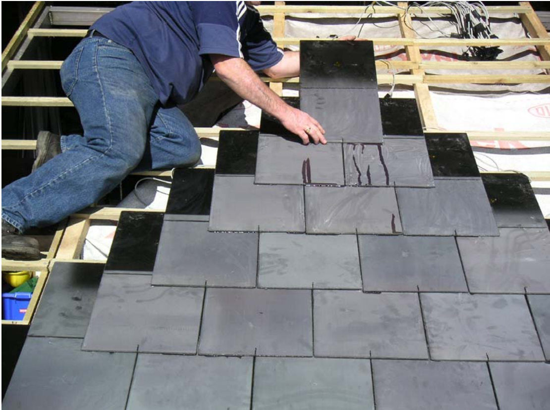
Fig BC. Demo Roof Installation work in progress.
