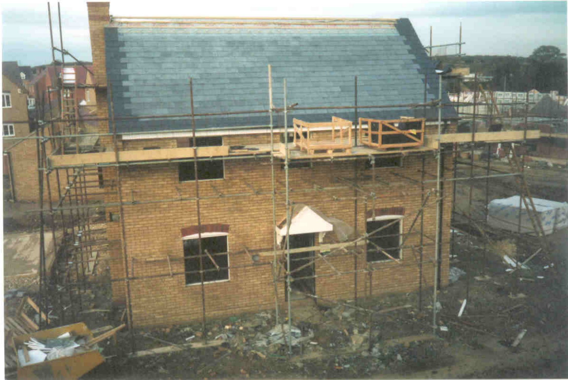
Fig F. Completed to ridge Level. View from Elevated Position.
