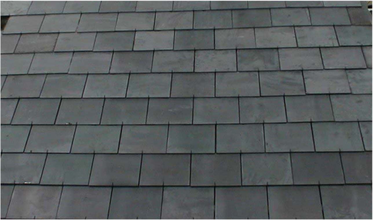
Fig BJ. Demo roof Section Completed.
