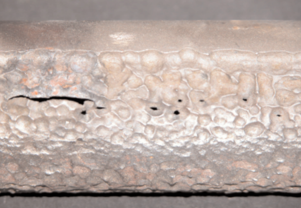
Figure 1. Superheater Tube Failure due to Fireside Corrosion
