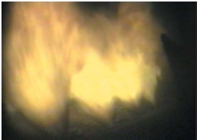
Figure 2. Oil burners in a corner fired unit during the start up sequence
