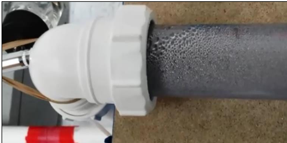
Figure 50: Liquid deposits in first portion of the pipe
