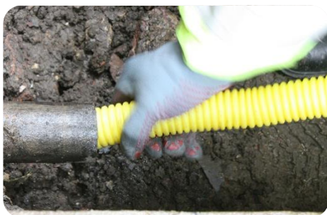
Figure 10: Serviflex pipe installation and with service head adapter fitted.
