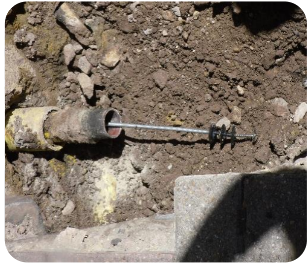
Figure 7: Show Inserting the sprung probe from the meter position. Figure 8: it arriving in the outside location service pit.
