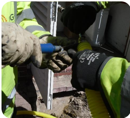
Figure 9: Fitting the flexible towing head to the end of the cut pipe length.
