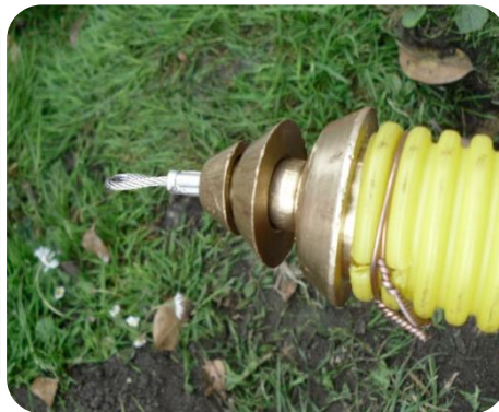
Figure 9: Fitting the flexible towing head to the end of the cut pipe length.
