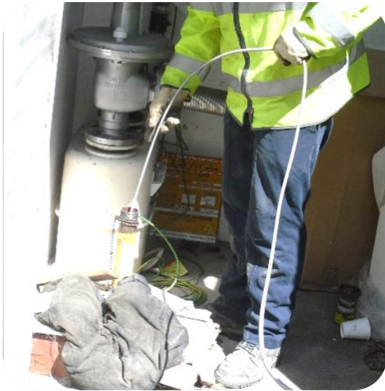
Figure 7: Show Inserting the sprung probe from the meter position. Figure 8: it arriving in the outside location service pit.
