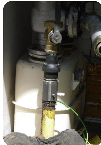
Figure 10: Serviflex pipe installation and with service head adapter fitted.
