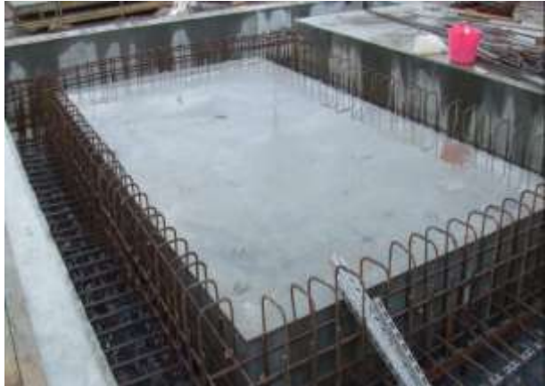
March – Concrete and rebar laid, foundations complete
