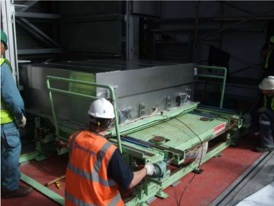
Figure 13 - Battery module insertion
