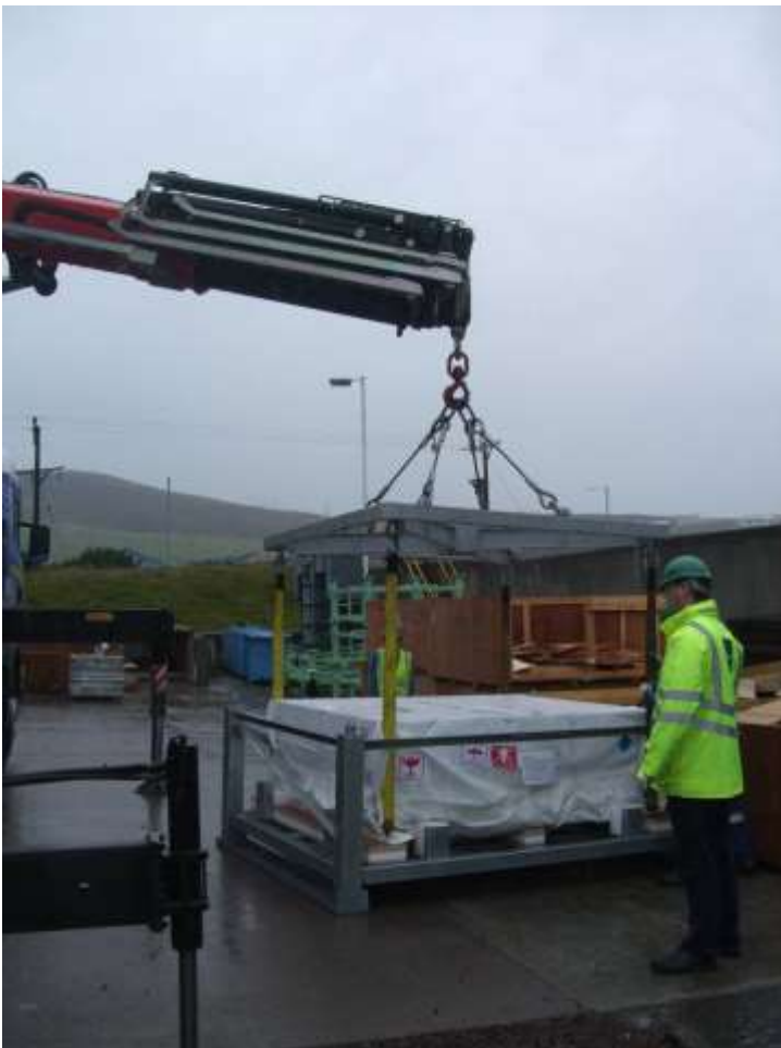
Figure 12 - Battery module being removed from transportation frame
