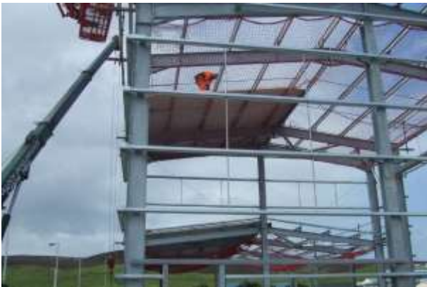
April – External building frame erected
