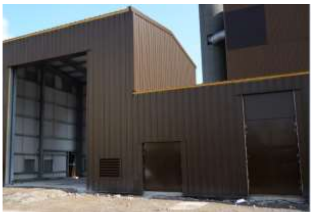
May – Building fully clad, internal works begin
