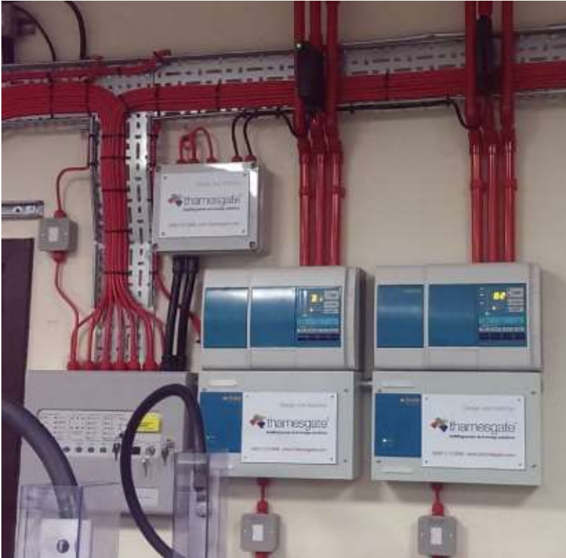
Figure 30 - VESDA and hydrogen detection
