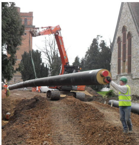
UK Heat Network Installation Galliford Try
