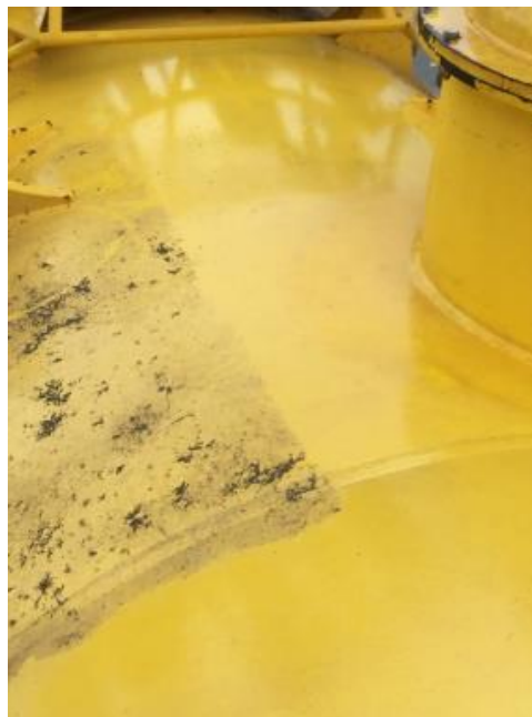
Figure 21 - Turbine nacelle showing areas before and after steam cleaning
