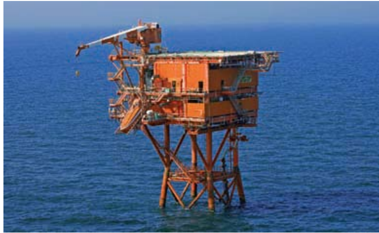
Figure 3-42: P18-A Satellite platform. (image courtesy TAQA; TAQA, 2009)
